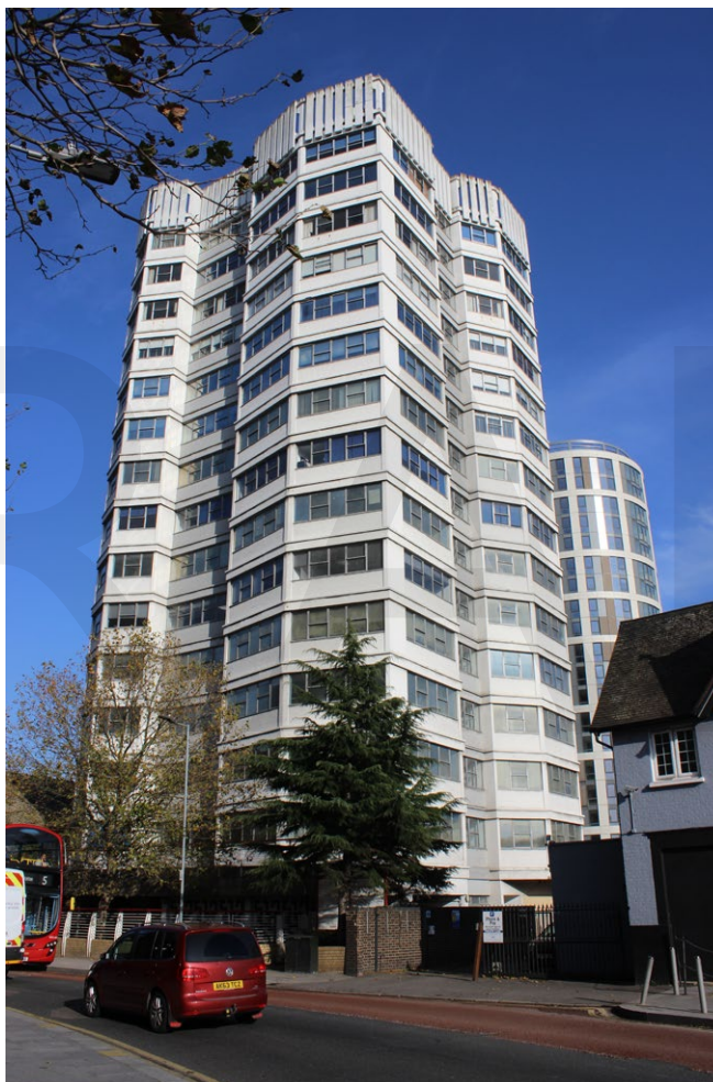
Crown House, Linton Road
